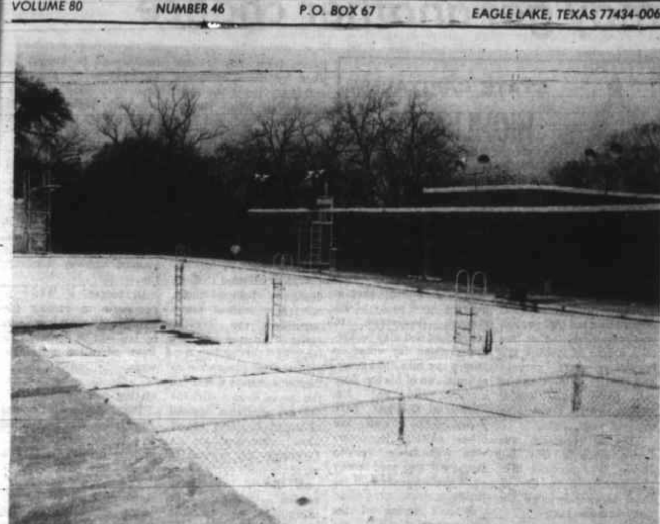
Swimming pool work begun
